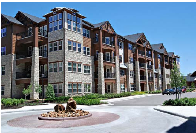
Example of 4-story multifamily Highlands Lodge, Overland Park, KS
